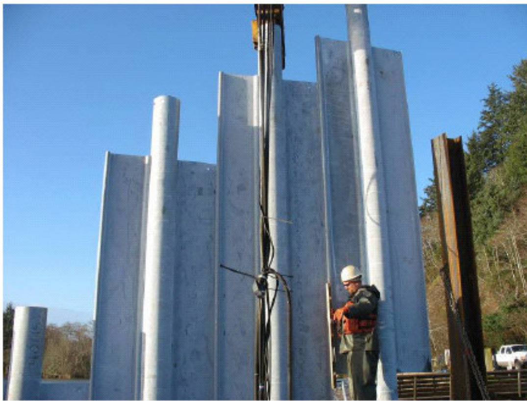
Figure 2: 12-inch diameter steel piles with interlocking 'wings' used to create the wave barrier (photo courtesy of Washington State Parks and Recreation, R. Johnson).
